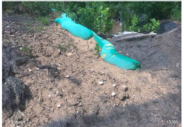
Figure 4: STA 13361+00 – CFS clean out needed.
