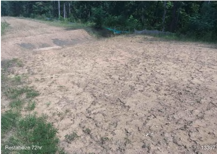
Figure 3: STA 13373+00 to 13371+00 – Re-stabilization needed.
