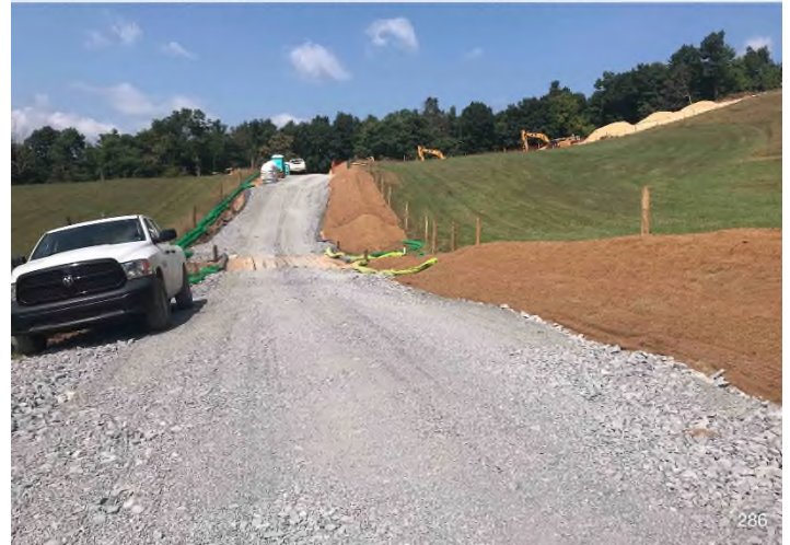
Figure 4: STA 12720+00 – Controls in place and functioning properly. Area stabilized with erosion control matting.
