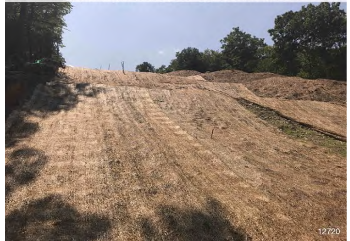
Figure 4: STA 12720+00 – Controls in place and functioning properly. Area stabilized with erosion control matting.
