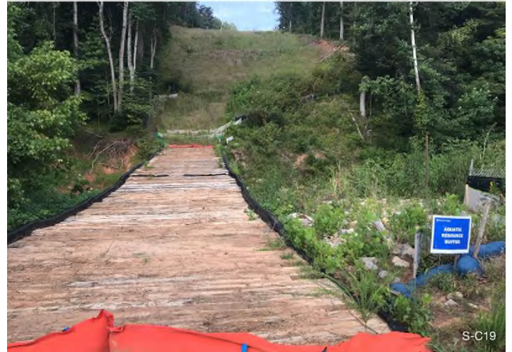
Figure 4: STA 14006+00 – Controls in place and functioning properly.
