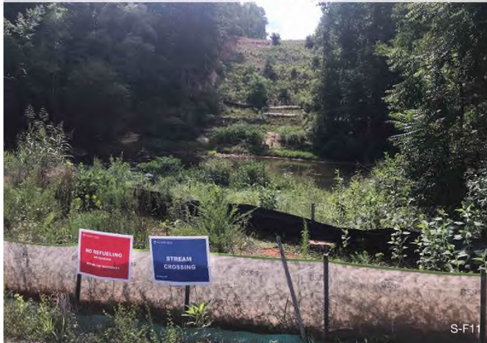
Figure 3: Stream S-F11 – Controls in place and functioning properly around Blackwater River crossing.
