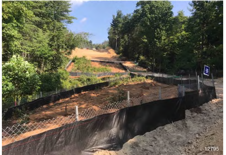
Figure 4: STA 12795+00 – Controls in place and functioning properly. Buffer established around S-IJ82.
