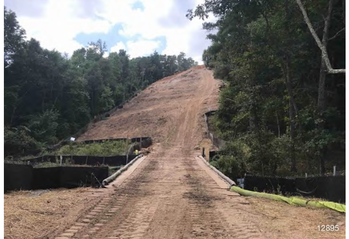
Figure 4: STA 12780+00 – Controls in place and functioning properly. BRG: 177°S (T) LAT: 37.174147 LON: -80.139134 ±16ft ALT: 2828ft
