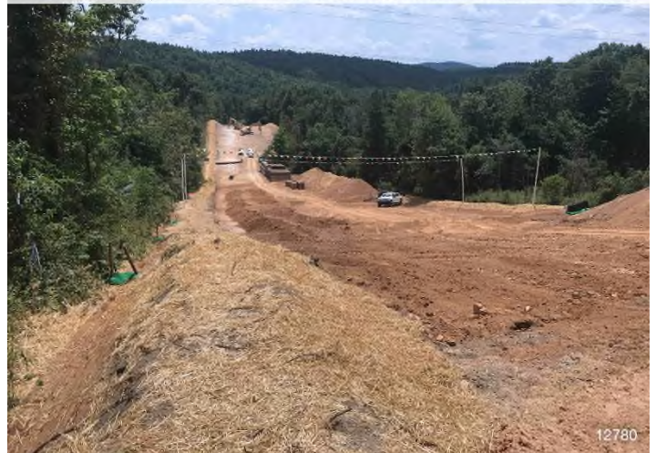
Figure 4: STA 12780+00 – Controls in place and functioning properly. BRG: 177°S (T) LAT: 37.174147 LON: -80.139134 ±16ft ALT: 2828ft
